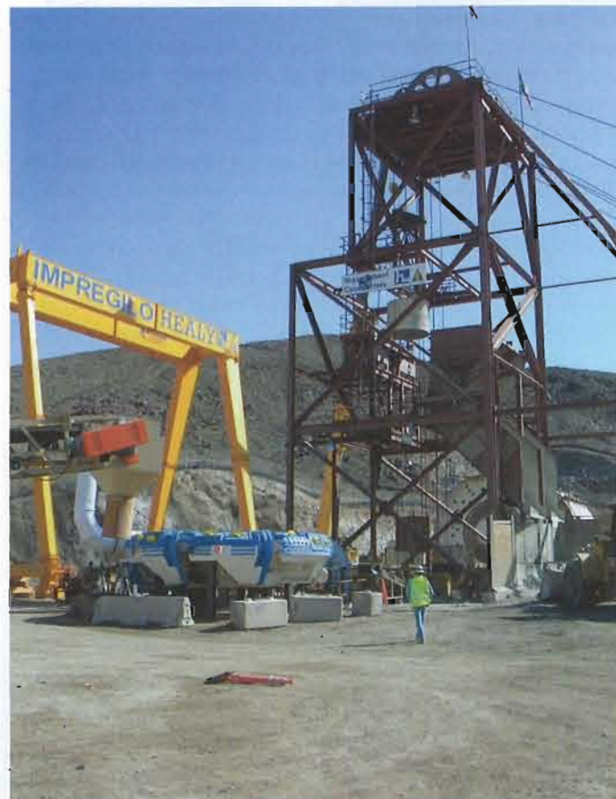
» Vegas Tunnel Constructors is digging a 600-foot shaft and will use a specialized Herrenknecht tunnel-boring machine designed to operate in high water pressure to drive the three-mile tunnel. The intake structure will be constructed on a barge at the shoreline and then lowered into a hole created by the use of explosives.
